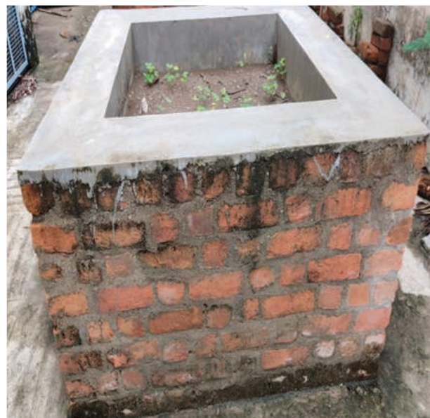
Fig. 1 (b) deep pit design for sanitary pads
